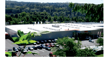
Coop Bau & Hobby, Winterthur, Suiza
