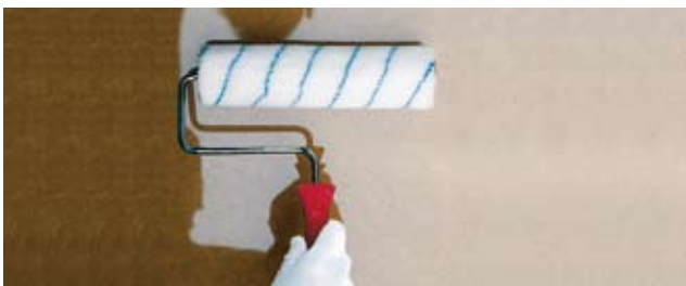
Primer application with medium pile roller.
