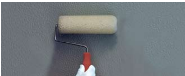
Application of Sika®-264 Thixo high build coating with a textured roller.
